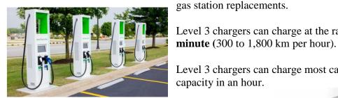
Level 3 chargers can charge at the rate of 5 to 30 km per
